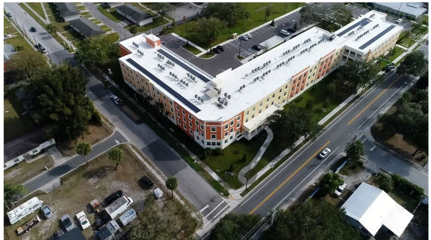
Amaryllis Park Place, 1912 N. Orange Ave., opened in February and was already full by mid-March – with a waiting list of about 50 people. Dan Minor
