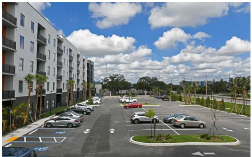
Lofts on Lemon is located at 750 Cohen Way, in Sarasota. A companion development, Lofts on Lemon II is also in the works on the same property. THOMAS BENDER/HERALD-TRIBUNE
