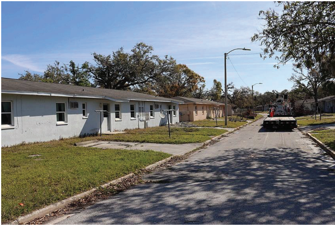
The Courts is being demolished to be replaced by future phases of Sarasota Housing Authority's Cypress Square.
